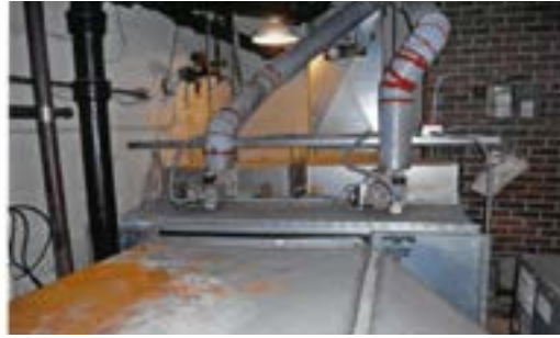
Furnace Room Before GBP
