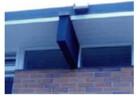
Beam Ends After GBP
